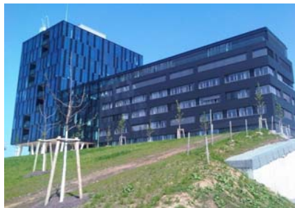
Karlsruhe, Park Office AG: Baresel GmbH, Osnabrück
